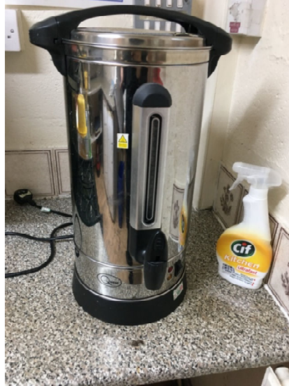
Photographs 6: Electric Point of Use Water Heater
