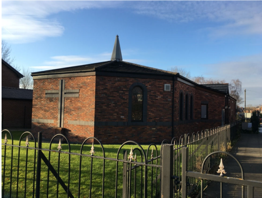
Photograph 1: Holy Angels Church External View
